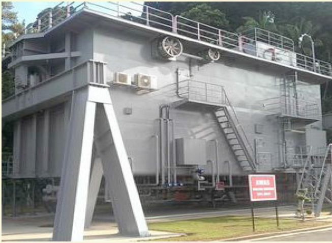
Fasiliti Damage Control Training Unit (DCMU)
